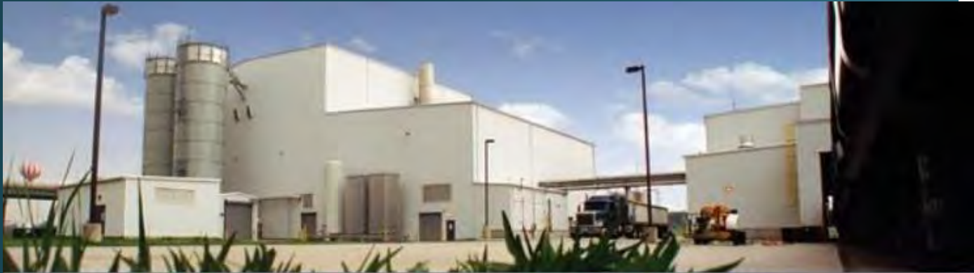
Sludge Drying and Pelletizing Plant - Chicago
